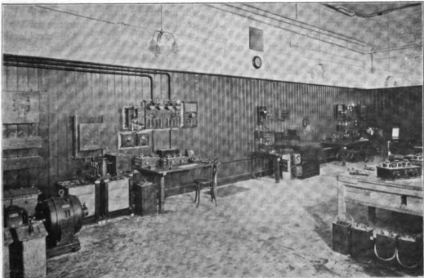
The Instrument Room, showing (from left to right) a 5-kw. Station, \frac{1}{2} -kw. Station, and 1\frac{1}{2} -kw. Station
