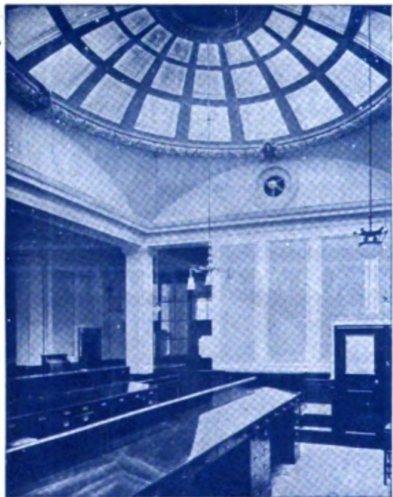
REINFORCED CONCRETE CUPOLA At Union of London and Smith's Bank, Hull.
